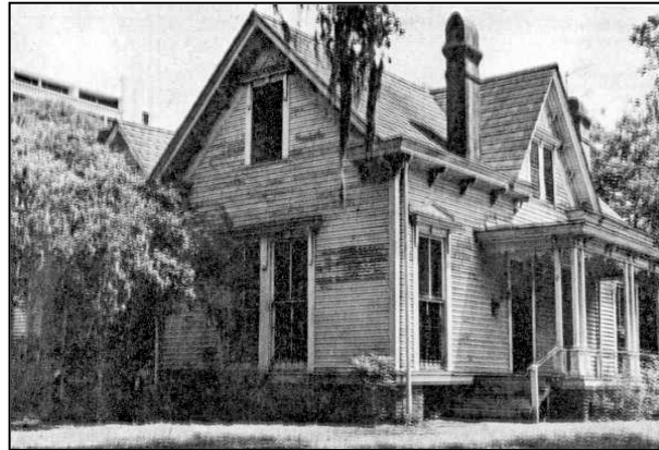
Cobb House at 403 North Calhoun Street 6
